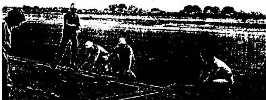
Fig. 16.15 (b) Application of geotextile in the main runway of the ahmedabad airport for prevention of reflection cracking
