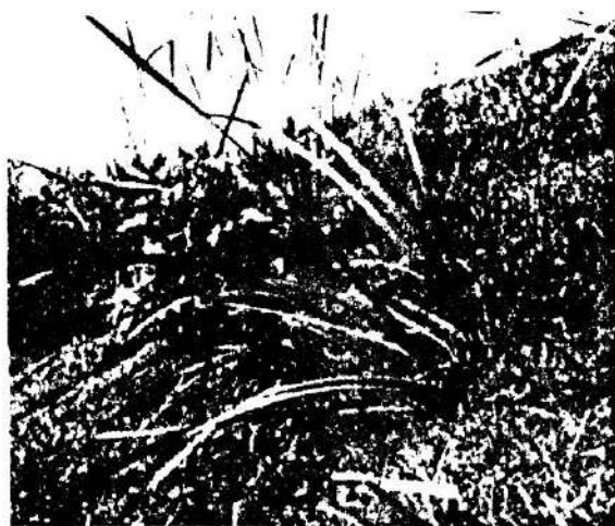
Fig. 16.9b Embankment slope covered with vegetation after protected with coir-netting
