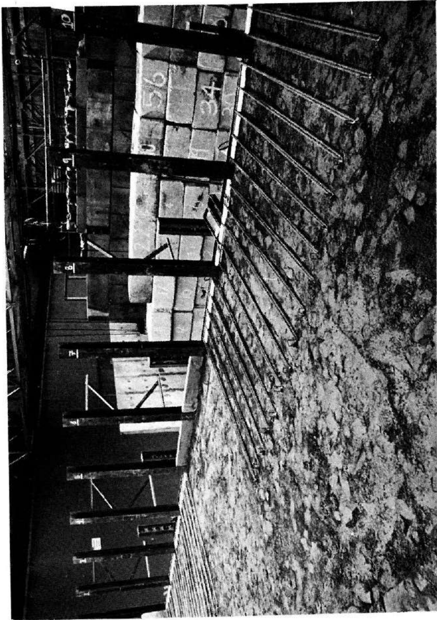
Arrangement of Rope Reinforcements Plate 4
