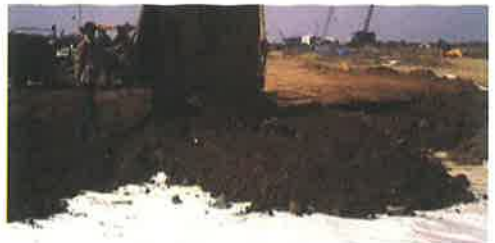
Morum Layer Being placed over Geotextile
