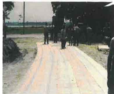
JGT LAID ON THE SUB GRADE
