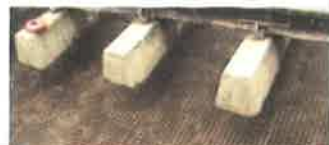
8 Laying TechGrid TGB-40 Knitted Polyester Biaxial Geogrid
