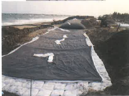
Photo2. Spreading of geotextile tube in position
