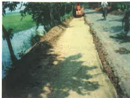
Photo 1. JGT laid over subgrade
