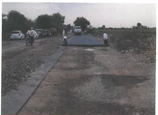
Unrolling TFI-5300 in 5m Widths
