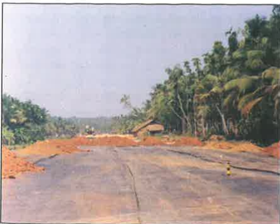
Installation of Techfab TPP 250 Woven Geotextile – Calicut Bypass , Kerala
