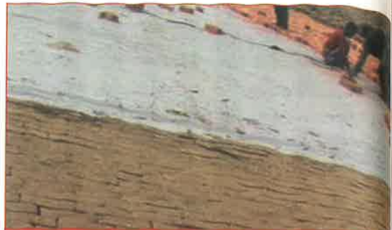
Unrolling of TechGeo Nonwoven Geotextile
