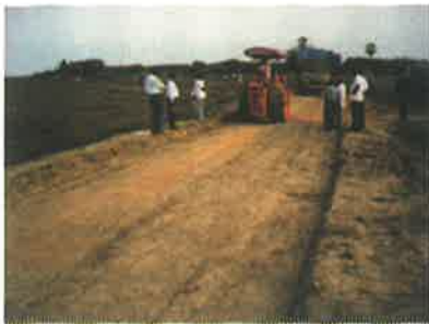
Fig.6. Finished subgrade
