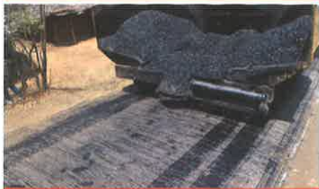
Over lay being laid over the TechGlass
