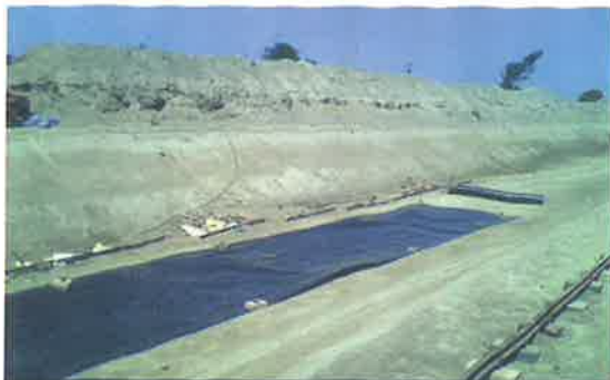
Photo 4 Unrolling & Laying of Drainage Composite
