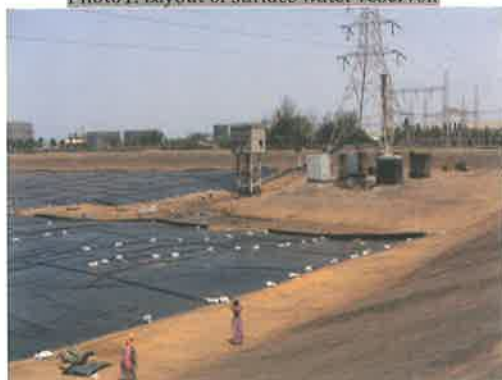
Photo2. Installation of HDPE geomembrane on bed
