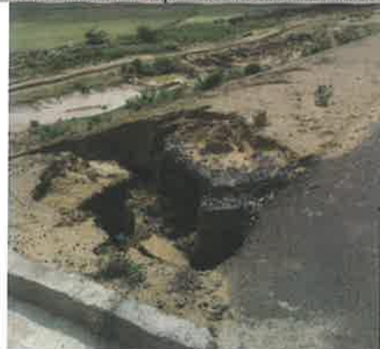
Photo2. Rain cuts on slope - before installation of Garmat®
