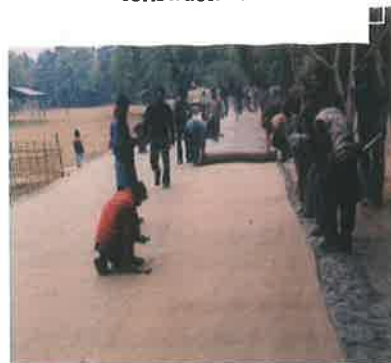
Photo 2. Laying of Jute Geotextile
