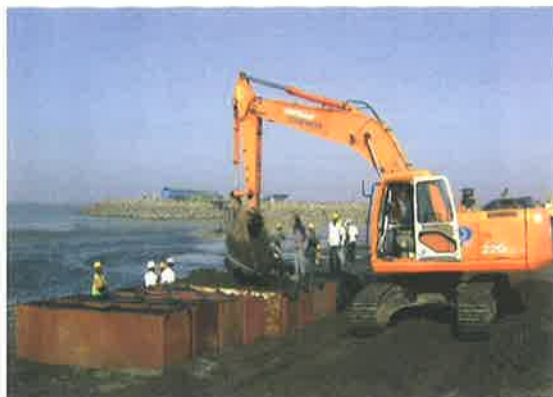
Photo2. Steel frames to support geotextile containers
