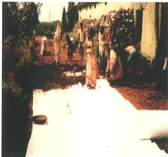
Laying of Geotextile
