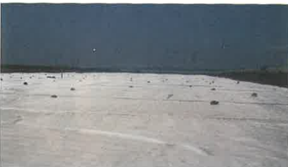
Photo 3. Placement of Basal Reinforcement over Drainage Layer in progress.
