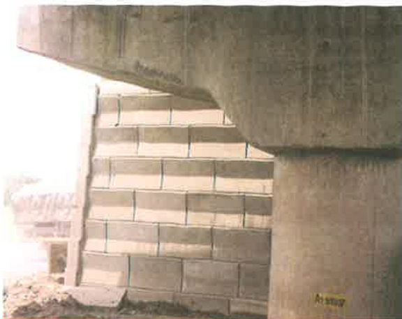
Abutment of RS Wall
