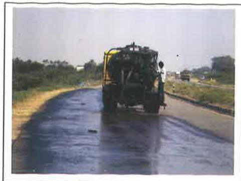
Tack Coat application on the existing pavement surface
