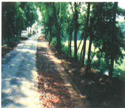
Photo 2. Brick metal laid over JGT
