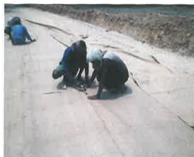
Photo 2. Stapling of Laid Jute Geotextile over Subgrade
