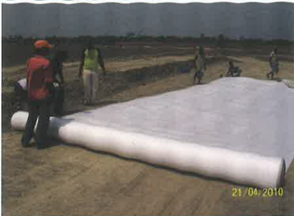
Photo 4 Unrolling Geotextile
