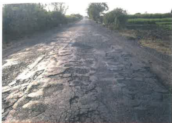
Distressed Pavement with Cracks
