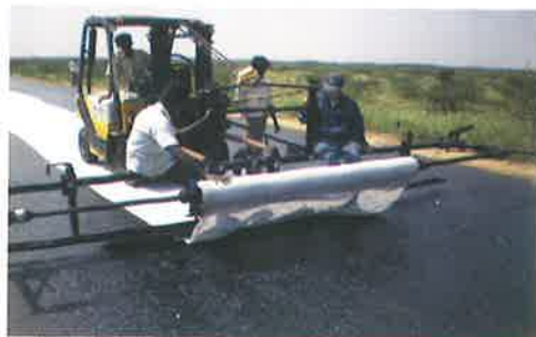
Paving Fabric rolled over using Mechanical rig
