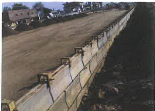
Erection of RS Wall
