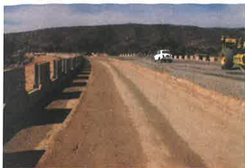
Erection of RS Wall
