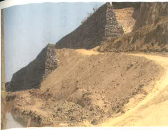
Picture 4. Two tier Gabion Retaining Wall after construction
