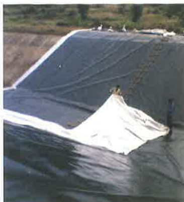
Photo 3. Installation of geomembrane and geotextile
