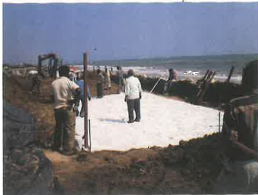
Photo1. Laying of geotextile and bags
