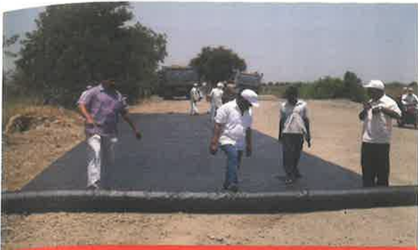
Laying of TFI-5300 at Subgrade
