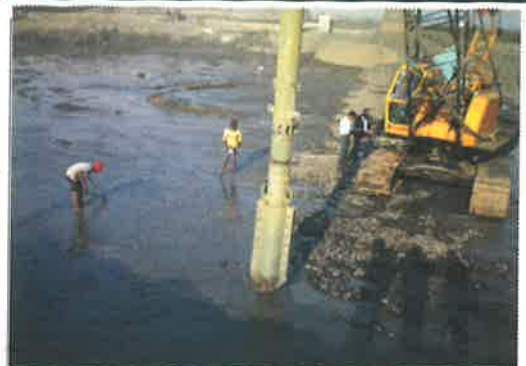
Photo 1 Installing stone columns
