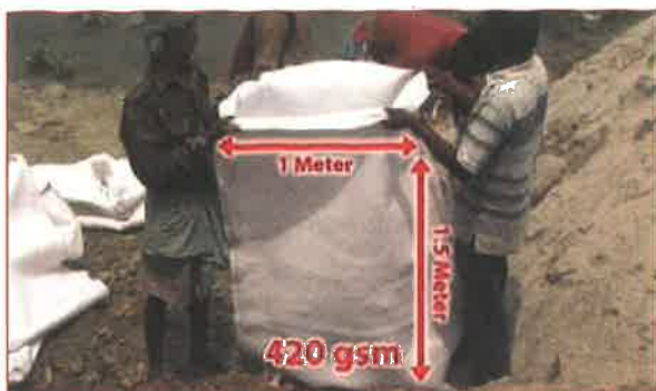
TechGeo Nonwoven Geotextile Bag Being Filled with Locally Available Fine Sand
