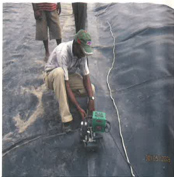
Photo 5 Joining of Geomembrane by wedge welding method
