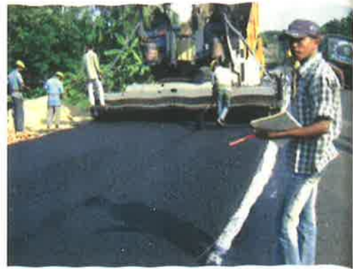
Paving with asphalt concrete
