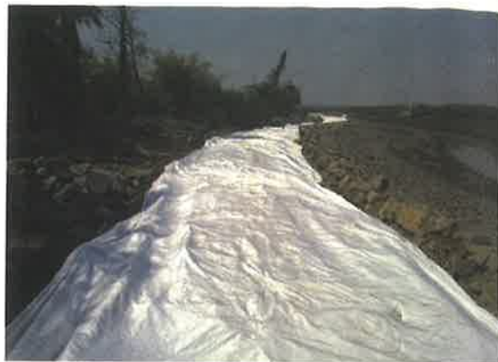
Laying of Geotextile
