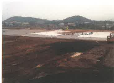
Photo 3. Construction of top liner system over geotextile stabilized layer
