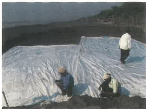
Laying of Geotextile
