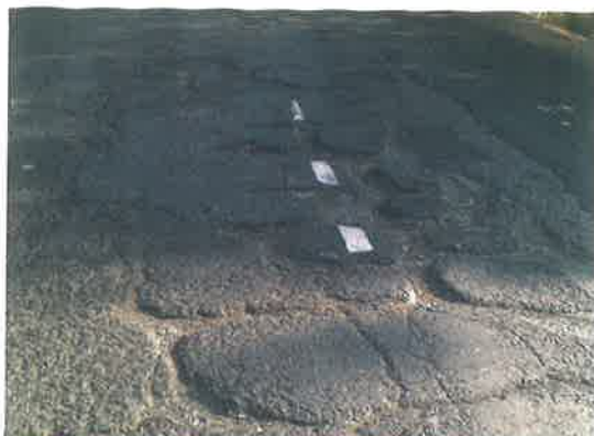
Photo 1 Before Construction—cracking on the surface
