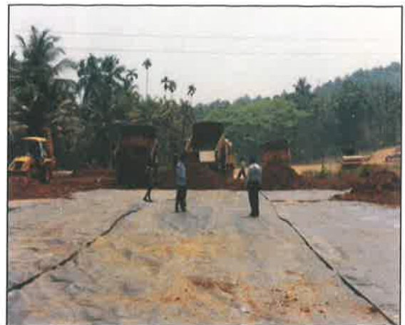
Installation of Techfab TPP 250 Woven Geotextile – Calicut Bypass , Kerala
