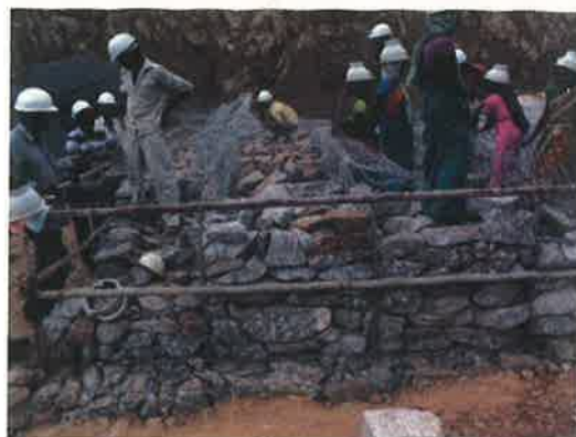
Picture 2. Filling of gabions with boulders
