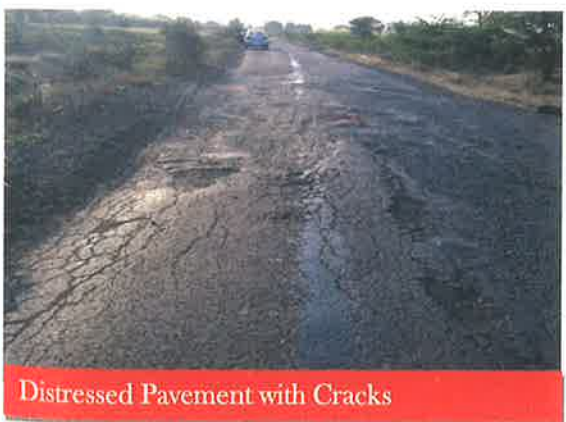
Distressed Pavement with Cracks
