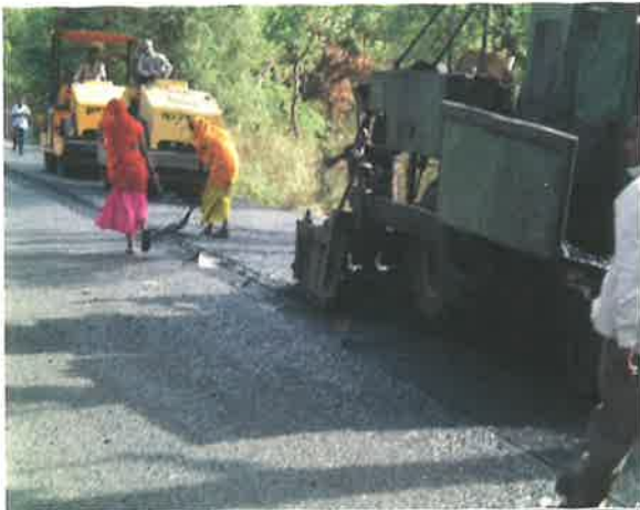
Photo 4 Laying of 20mm thick SDBC layer
