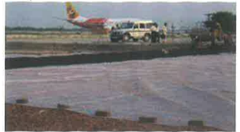
Installation of Secugrid 40/40 Q1
