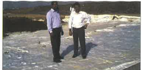
Laying of High Strength Geotextile TFI 3200
