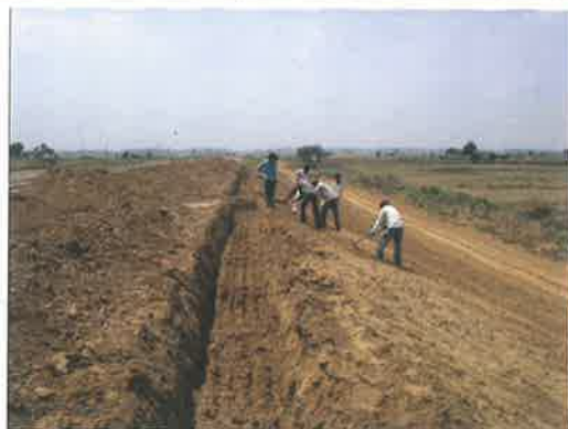
Photo3. Surface preparation in progress for installation of Garmat®
