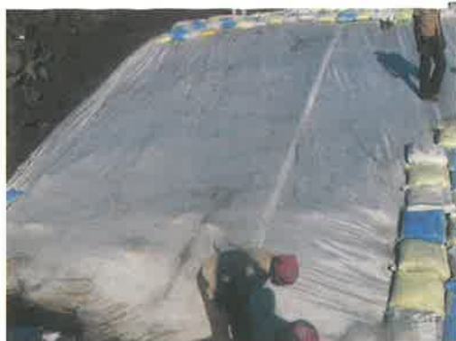
Laying Of Geotextile
