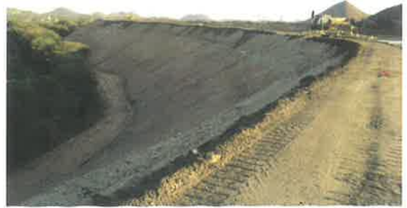
Photo5. Geotextile reinforced embankment after construction
