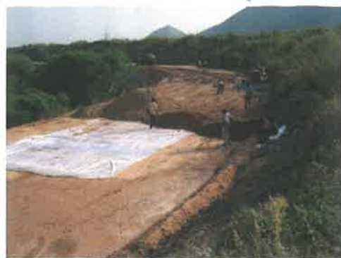
Photo2. Spreading of geotextile reinforcement in progress
