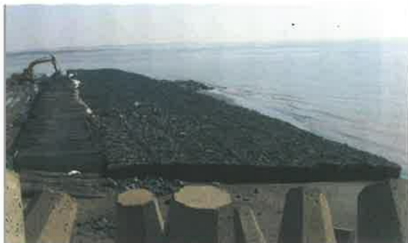
Photo1. Apron using PP rope gabions
