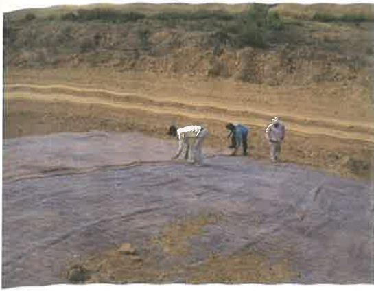
Photo4. Installation of Garmat® and soil placement in progress
