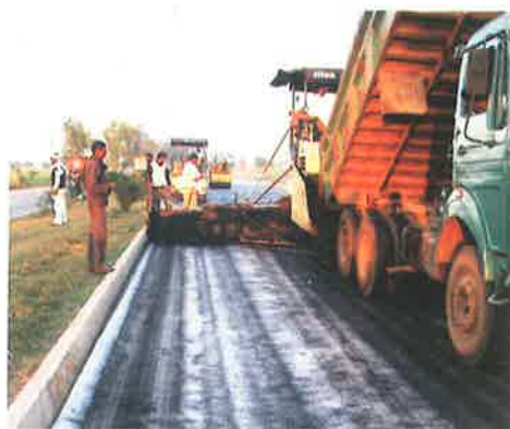
Asphaltic overlay installed on the Paving fabric
