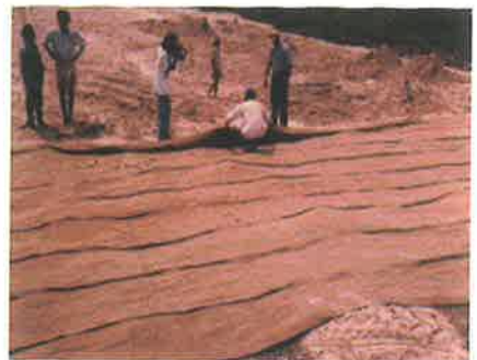
Photo 2. Laying of Jute Geotextile over Sand
