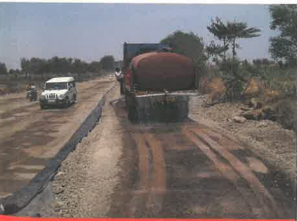
Sprinkling of Water & Compaction of Pavement
