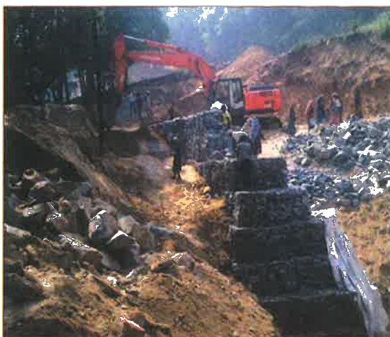
TechFab Metal Gabion Installation
