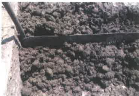
Geostrips used in joint cutting avoided
