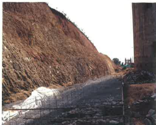
Picture 3. Construction of Gabion Retaining Wall in progress
