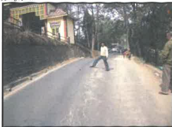
Settlement of 50cm on Valley-Side Pavement
