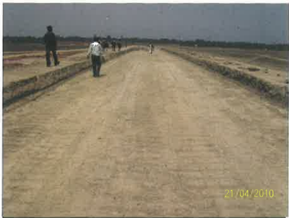
Photo 3 Embankment ready for laying Terram 2000
