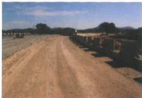
Erection of RS Wall
