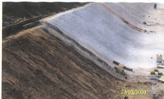
Photo 5 Placed Drainage composite at
