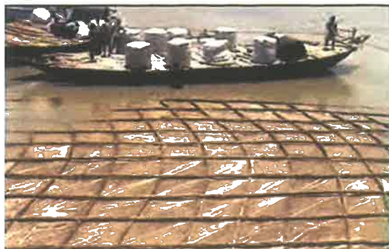
Laying of Woven Geo filter using Bamboo Strips
