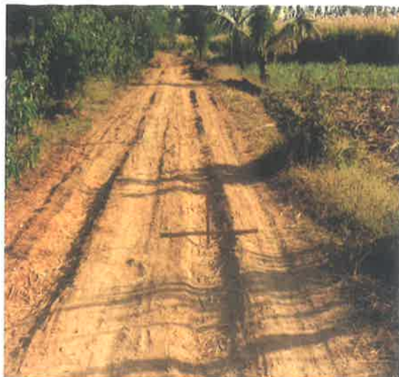
Rut on Road Without Geotextile
