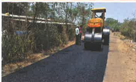
Compaction of Over Lay
