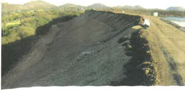
Photo4. Geotextile reinforced embankment, 14 m high after construction
