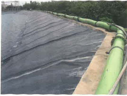
Photo4. Anchoring of geomembrane below the pipe line
