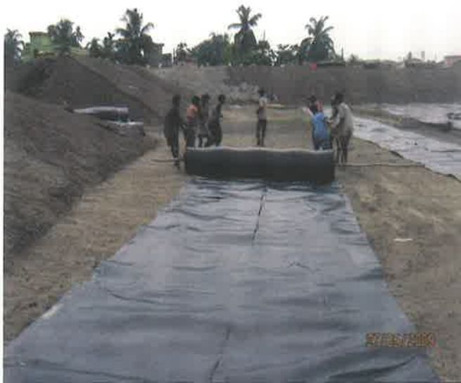
Photo 4 Unrolling & Laying of Geomembrane
