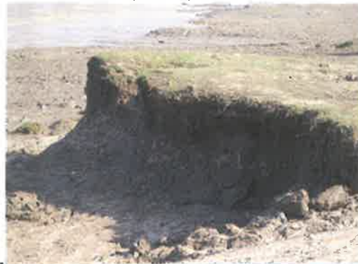
Photo 1 Site eroded due to wave effect
