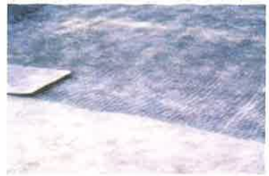
Laying of Techgrid U-40 as a basal reinforcement
