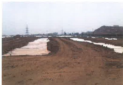
Photo 2. Construction of geotextile stabilized soil layer system over sludge using finger fill soil placement technique
