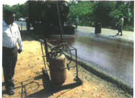
Spraying Tack Coat
