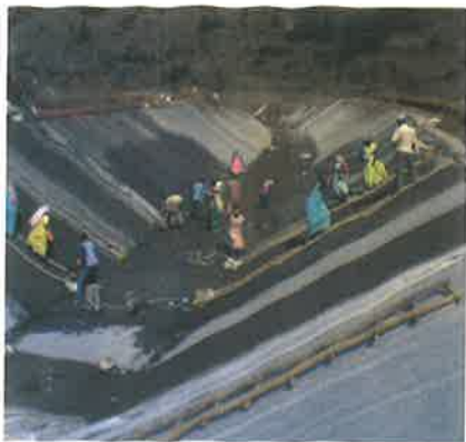
Photo4. Construction of top concrete layer
