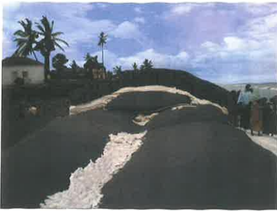
Photo4. Typical cross-section of geotextile tube sea wall (2 + 1 configuration) along with PP rope gabion as armour layer
