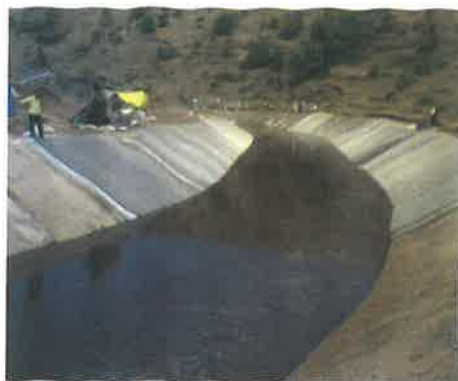
Photo5. Water flow in canal after completion of geomembrane lining
