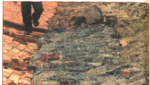
Metal Gabion Placed at Bottom Trench
