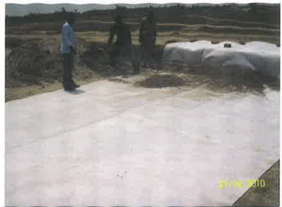
Photo 5 Sand Filling on Geotextile
