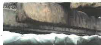
6 Laying of non-woven geotextile
