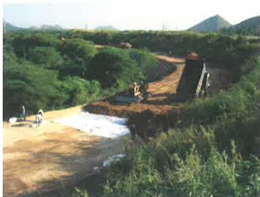
Photo3. Earthwork operations in progress over the geotextile reinforcement
