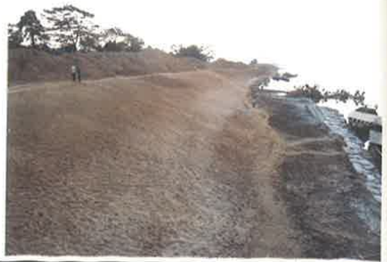
Photo 4 River bank dressed to 1V:3H slope
